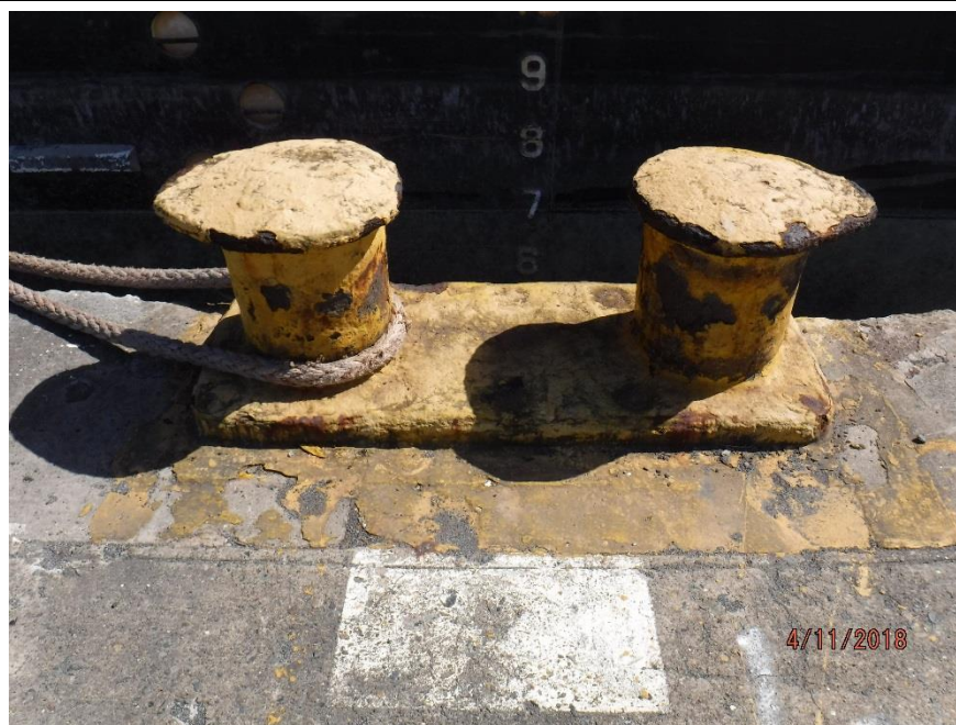
Photo 24. Wharf – View of a typical double bitt near Sta. 5+92.
