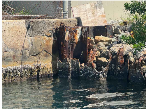
SHEET PILE WITHOUT CONCRETE CAP
