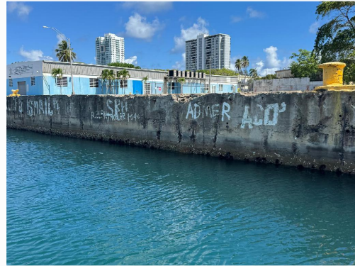
EXISTING BULKHEAD CONDITIONS
