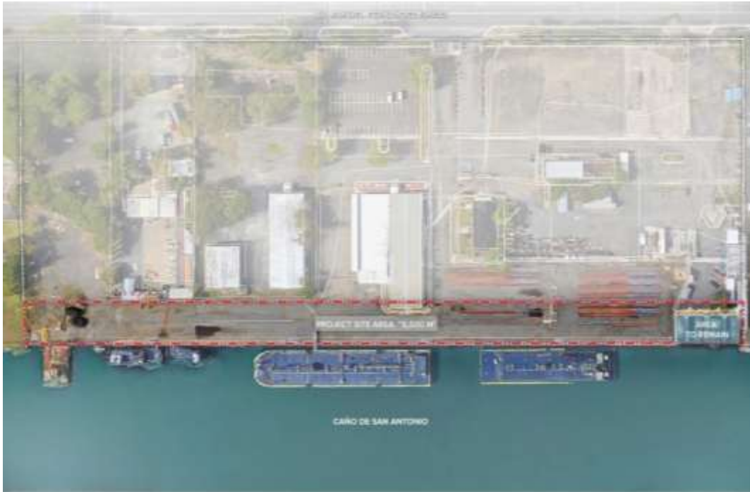
Figure 2- Aerial Image of the Navy Pier Bulkhead and Boardwalk Project
