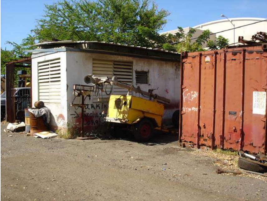
Picture 52. Partial view of the inspected areas.
