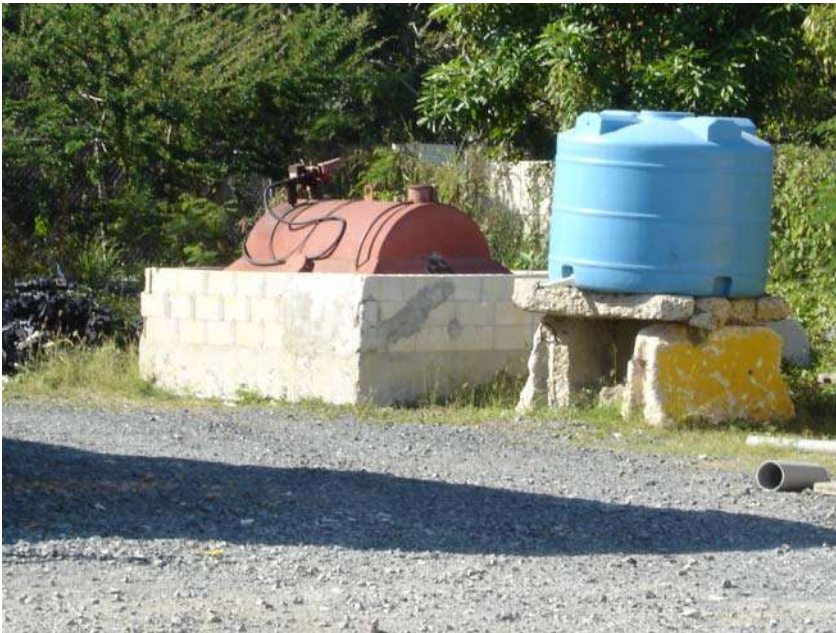
Picture 103. AST and Water tank.
