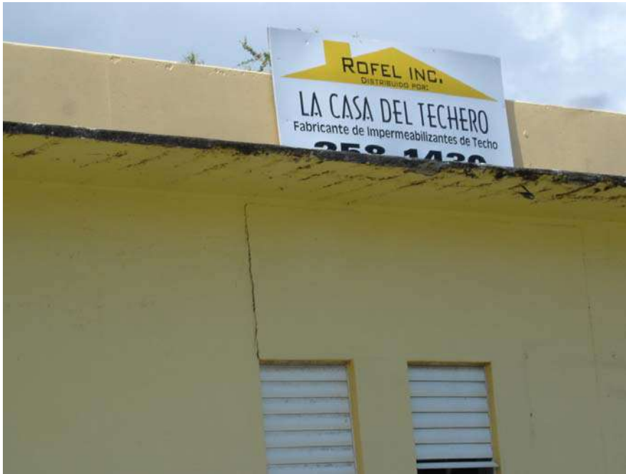
Picture 25. Main structure looking south.
