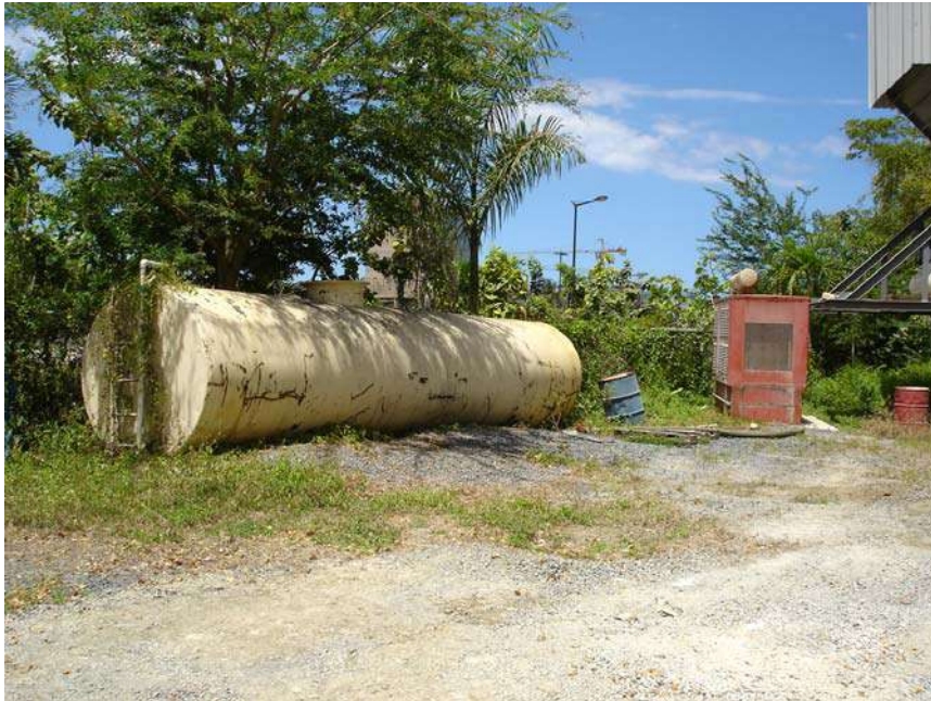
Picture 94. Abandoned AST and electric generator.
