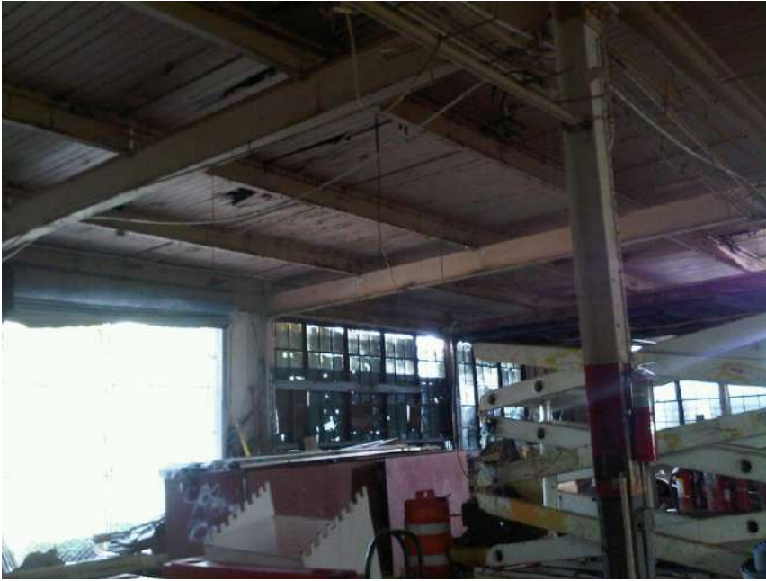
Picture 50. Interior view.
