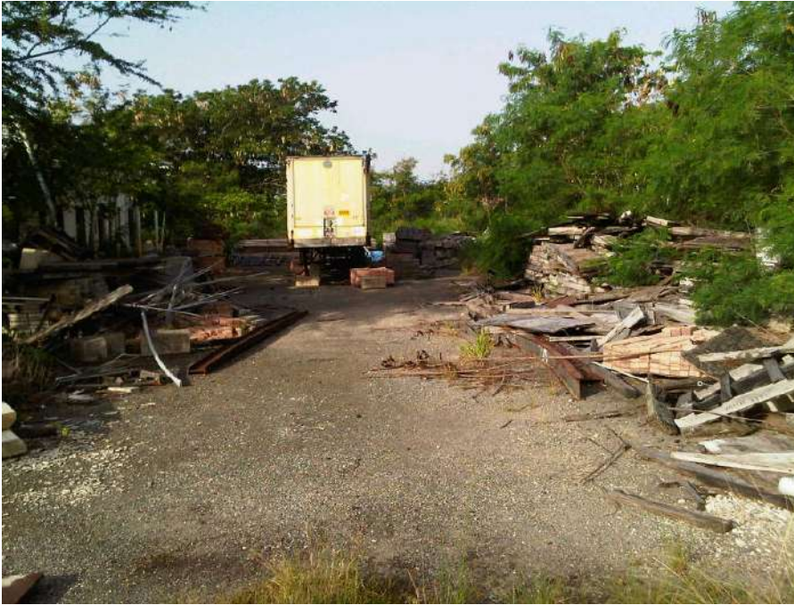
Picture 48. Significant accumulation of debris south of the main structure.
