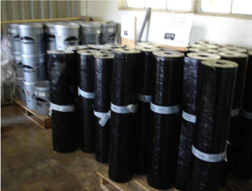
Picture 27. Roof sealing products storage inside the building.
