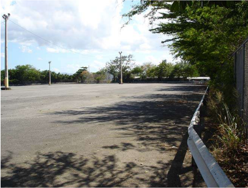
Picture 107. Site view looking southwest.
