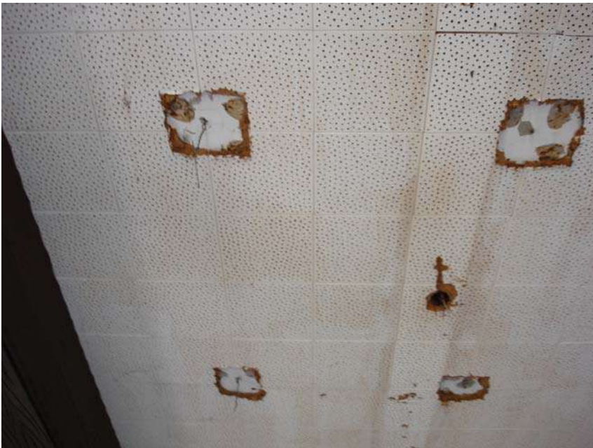
Picture 87. Ceiling tiles may contain ACMs.
