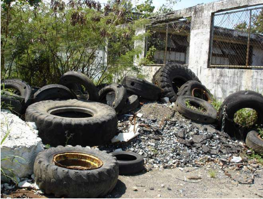
Picture 44. Solid waste accumulation north of the main structure.
