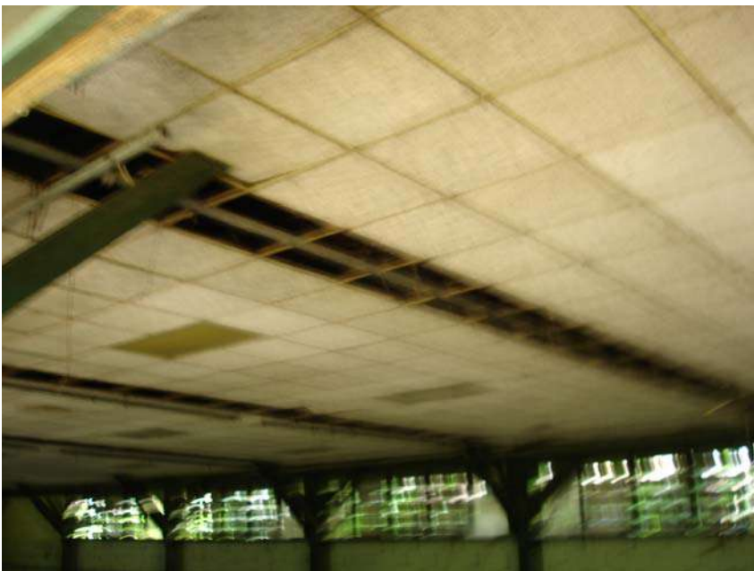
Picture 115. Structures at the site may contain ACMs in floor and ceiling tiles.
