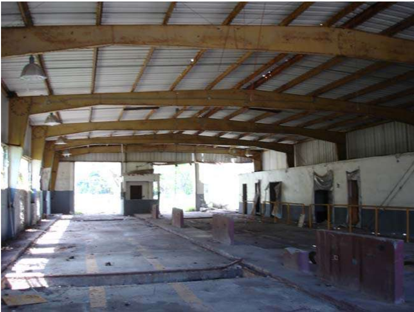
Picture 77. Interior of the structure.
