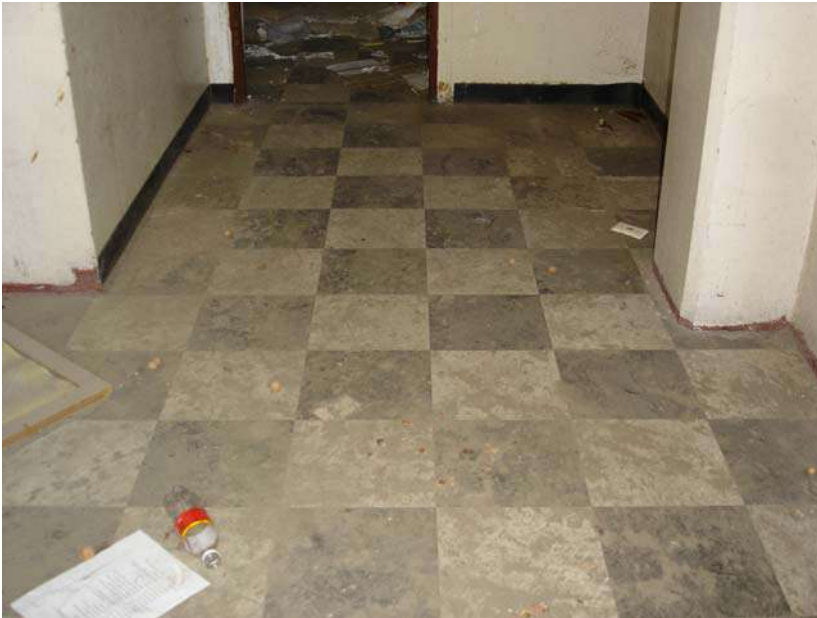
Picture 91. Vinyl floor tile at another location on the first floor.
