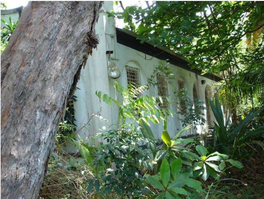
Picture 117. Structure consists of a single-story concrete building.
