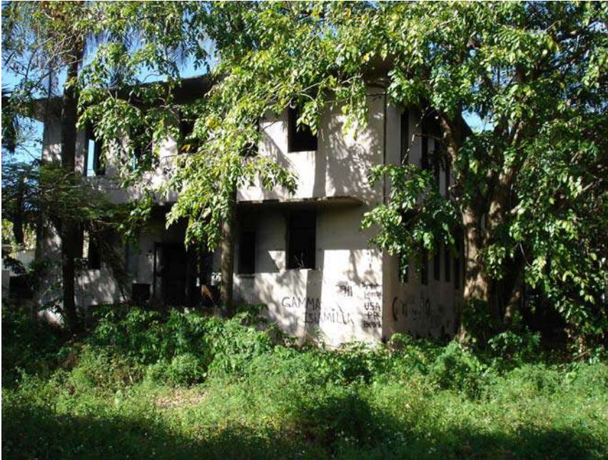
Picture 78. Main structure looking south.
