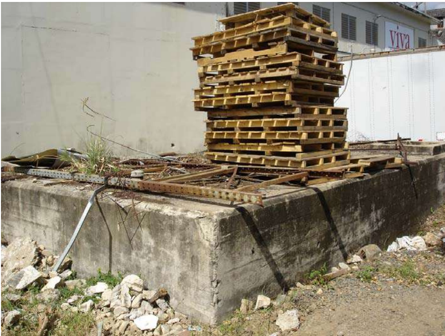
Picture 14. Concrete tank located north of the site.
