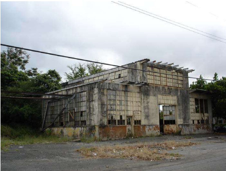
Picture 2. Side building looking west
