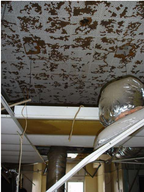
Picture 89. Ceiling roof tiles.
