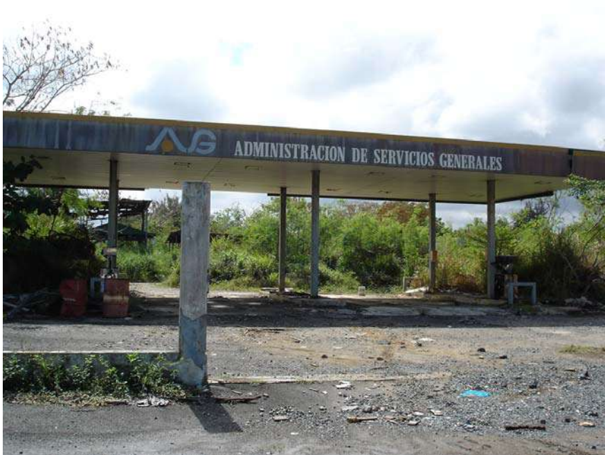
Picture 30. Main structure looking east.
