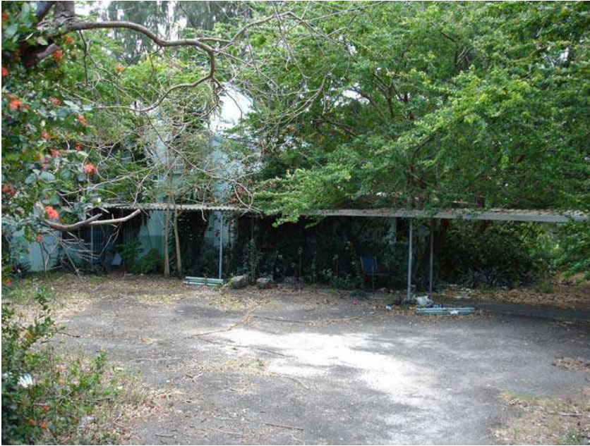
Picture 120. Main structure looking west.
