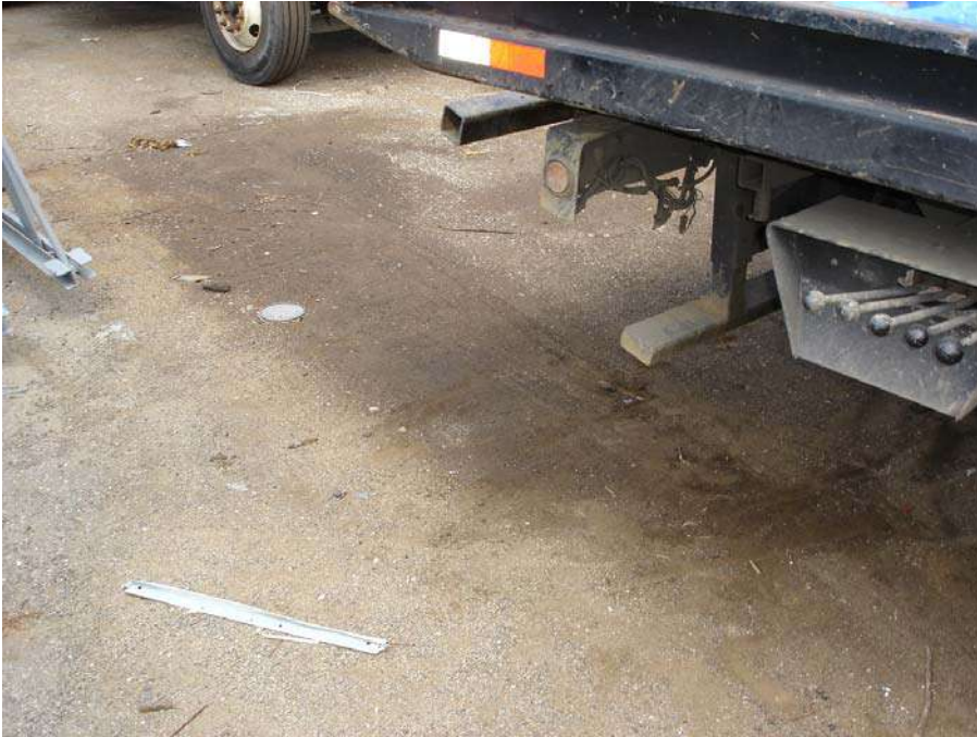
Picture 23. Oil stained asphalt observed close to the electrical sub-station.
