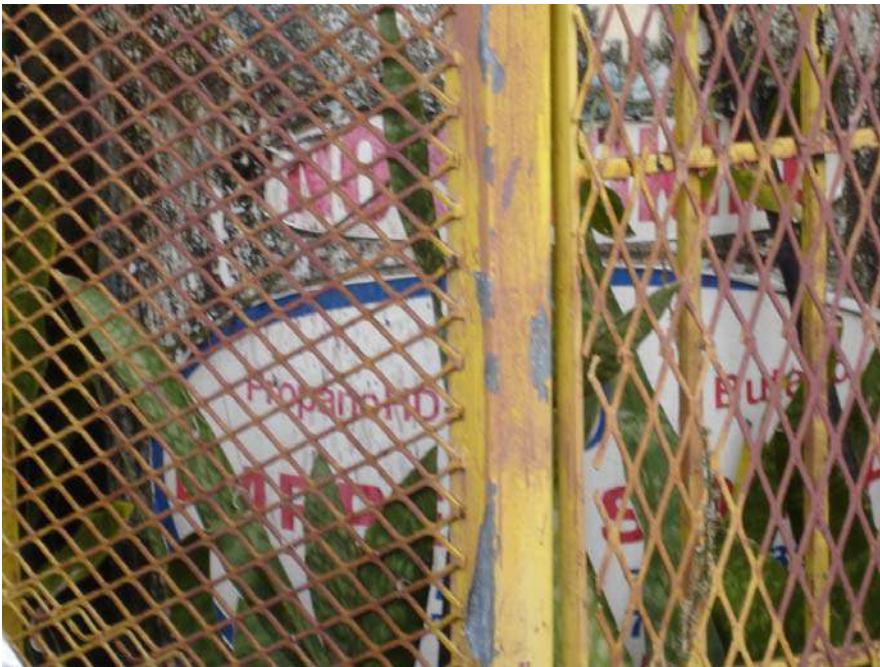
Picture 20. Propane Gas storage tank located south of the structure.
