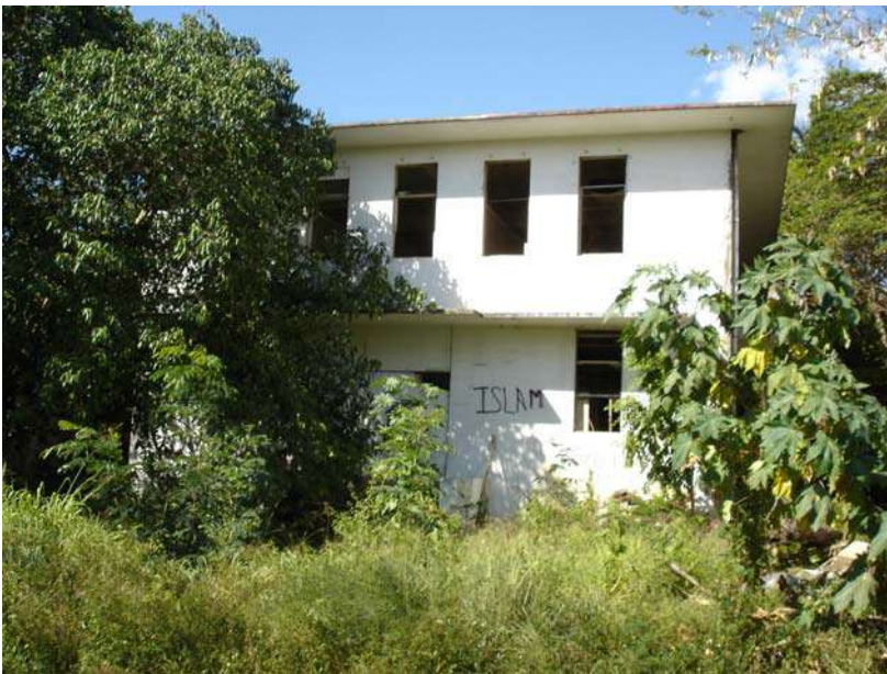
Picture 81. Front view of the site.
