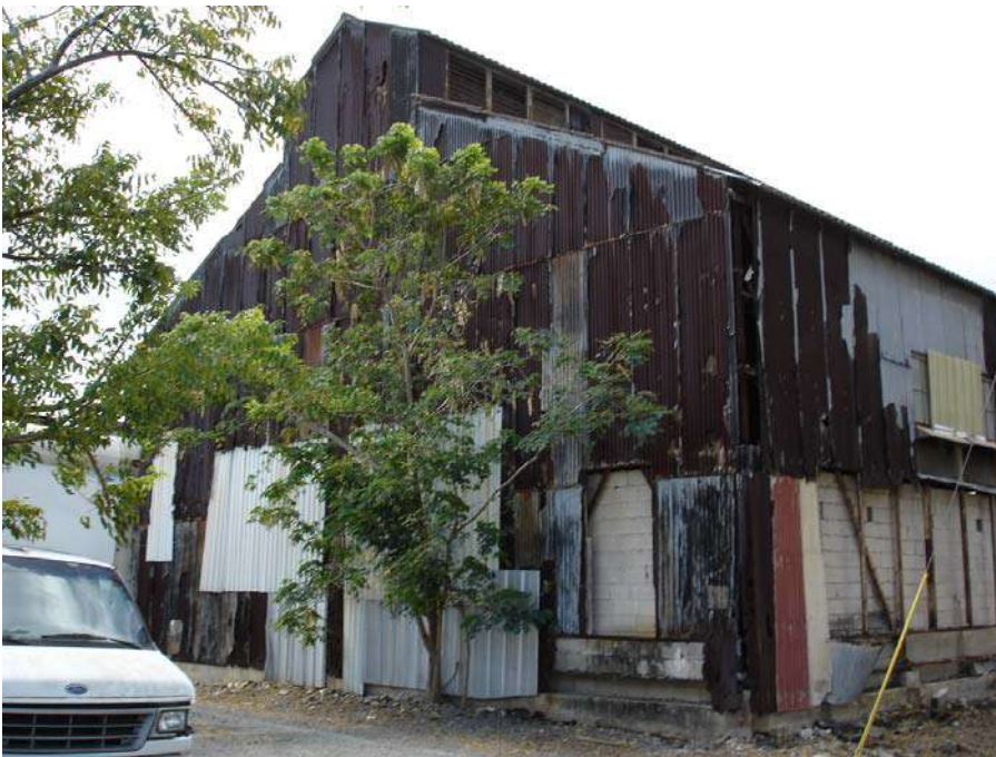
Picture 12. Annex building looking south.
