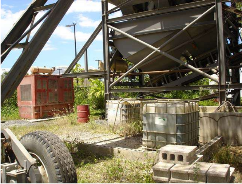
Picture 100. Concrete mixing plant.
