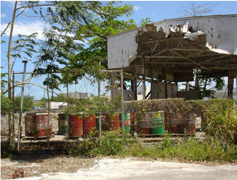
Picture 101. More than 70 55-gallon drums, mostly unlabeled are accumulated at the southeast corner of this site.
