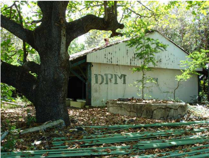
Picture 115. A concrete tank, purportedly used to store water, was documented at the site.
