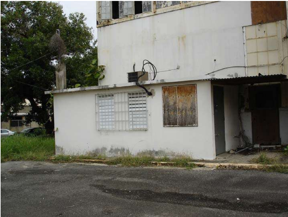
Picture 3. Annex building
