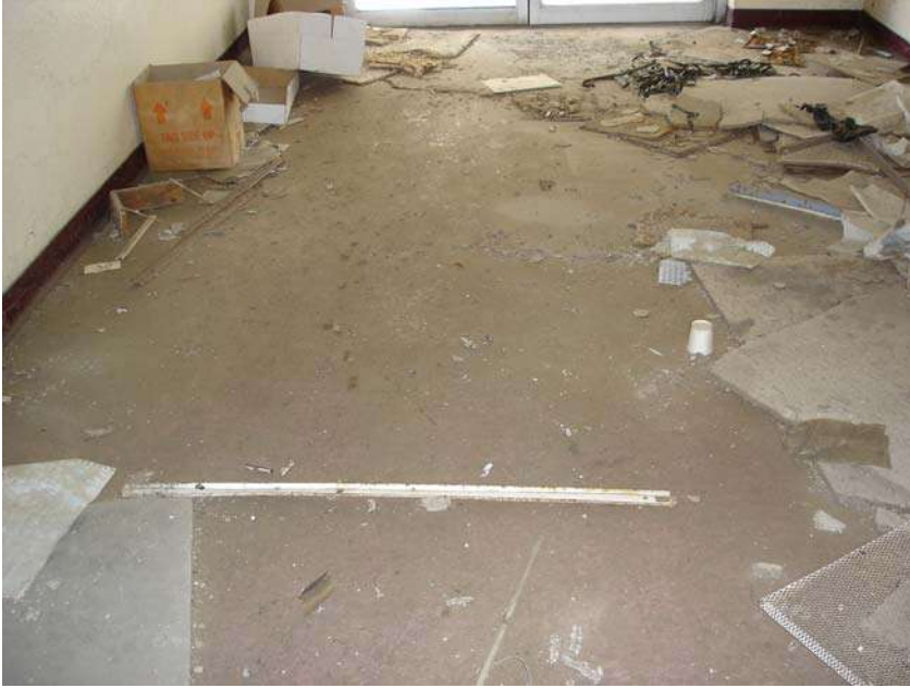
Picture 90. Vinyl floor tiles are present throughout most of the building.
