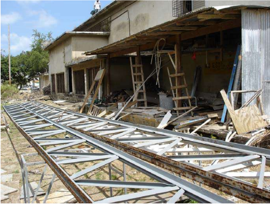
Picture 17. Another view of the main storage facility.
