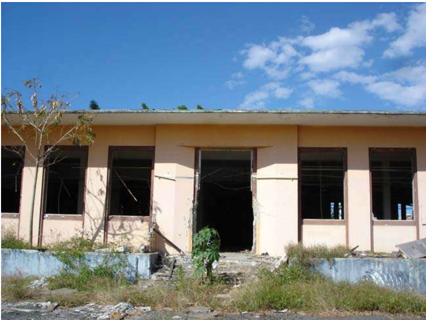
Picture 85. Main structure looking north.
