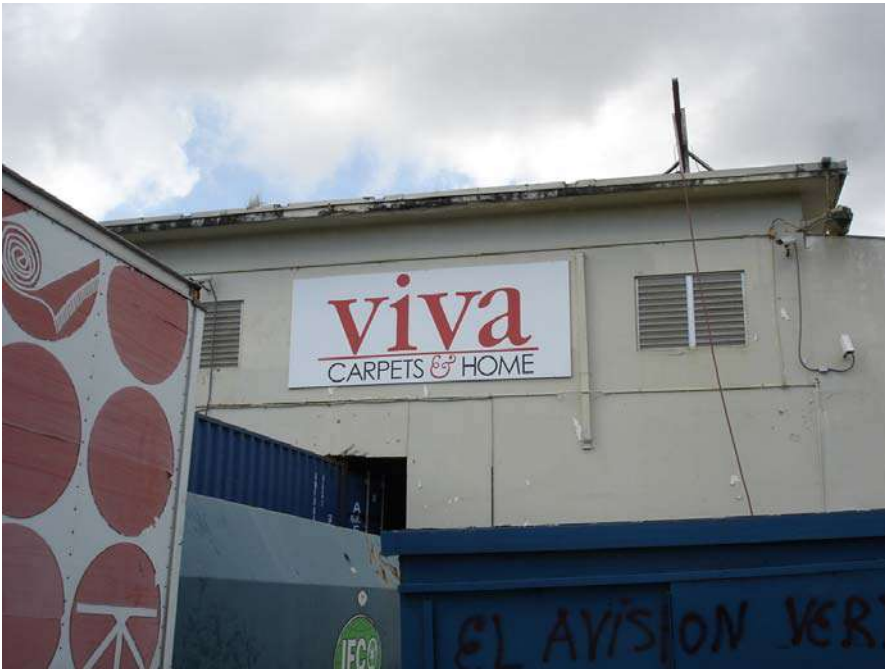
Picture 8. Main structure looking south.
