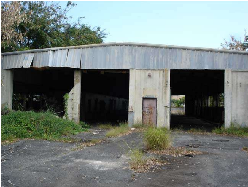
Picture 75. Main structure looking north.
