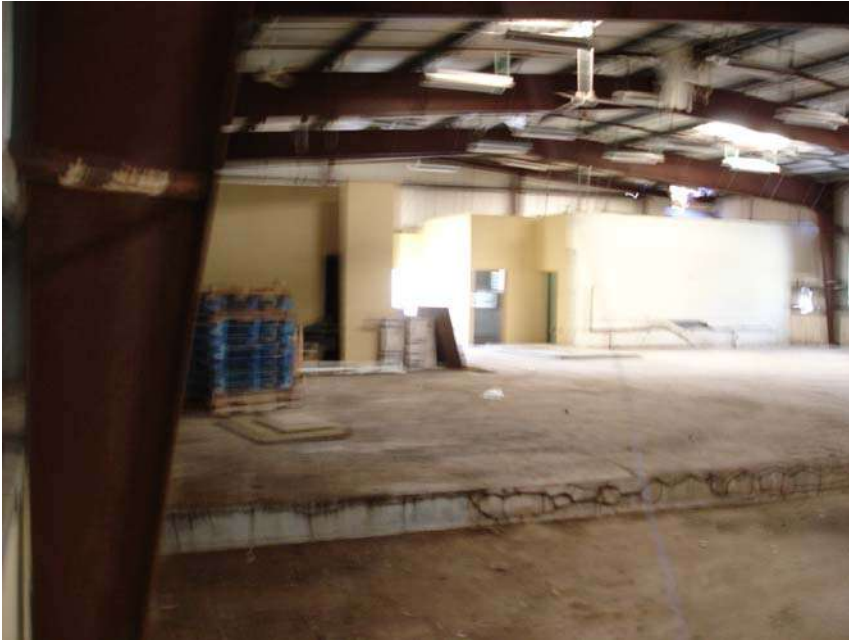
Figure 68. Wood pallets can be observed east of the building.
