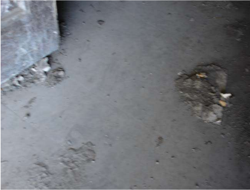
Picture 80. Vinyl floor tiles may contain ACMs.
