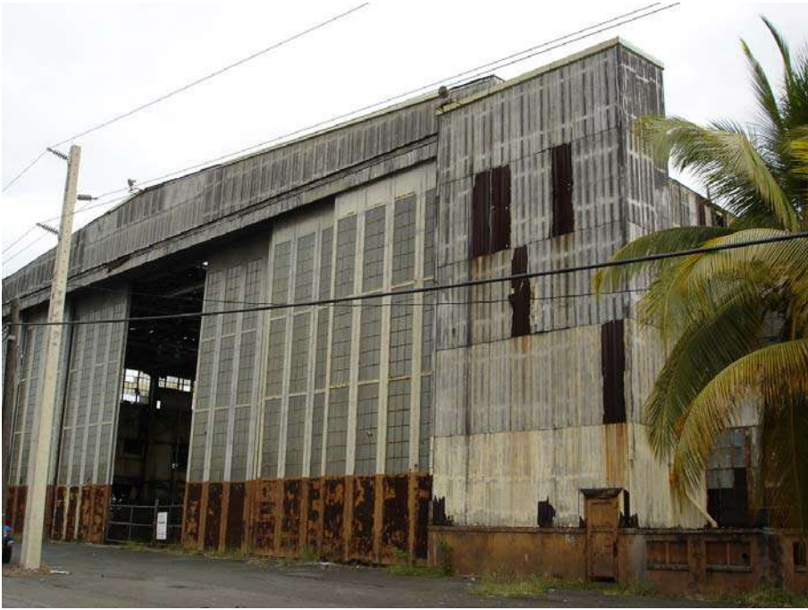
Picture 1. Main structure looking north.
