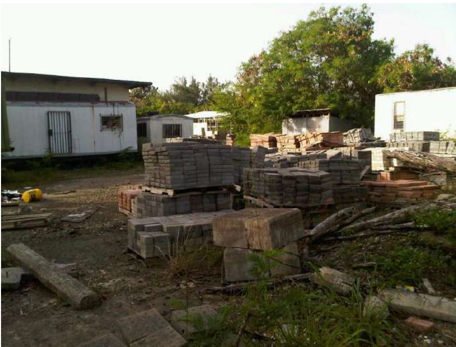
Picture 49. Alternate view of accumulation of debris south of the main structure.
