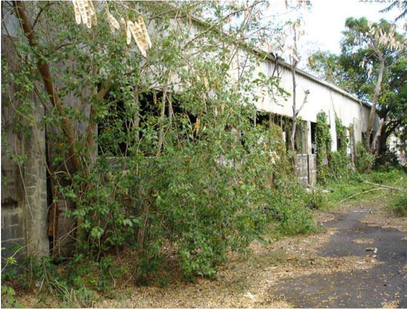
Picture 76. West side of the main structure.
